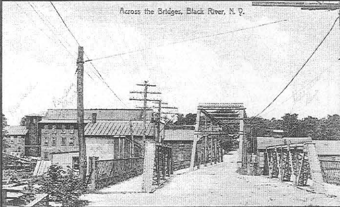
Across The Bridges, Black River, NY
