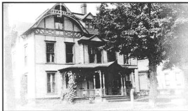
A picture of a building found among the unidentified Johndrow pictures
