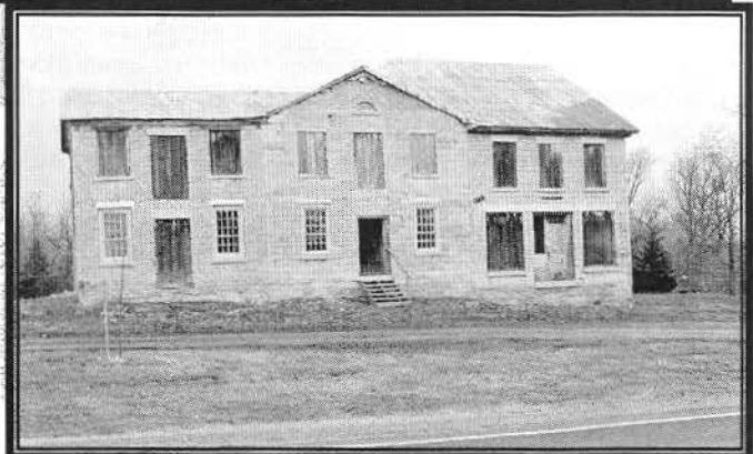
Renovations being done today (March 2007) on the store - See Page 21 for old picture of store
