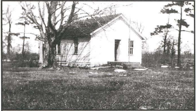
Lee School #5 Depauville-Brownville Rd near VanAlstyne Rd
