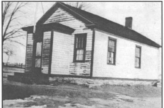
Green Settlement District School #10
