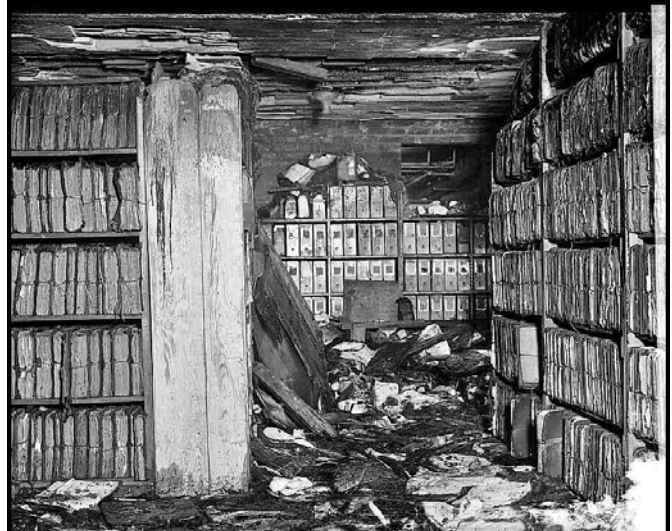
Storage area inside the Commerce Building after the 1921 fire (from the National Archives)
